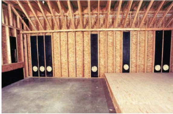
Shown above is the same CAT project with room balancing subwoofers (RBS); the project is also equipped with an SBMS.
